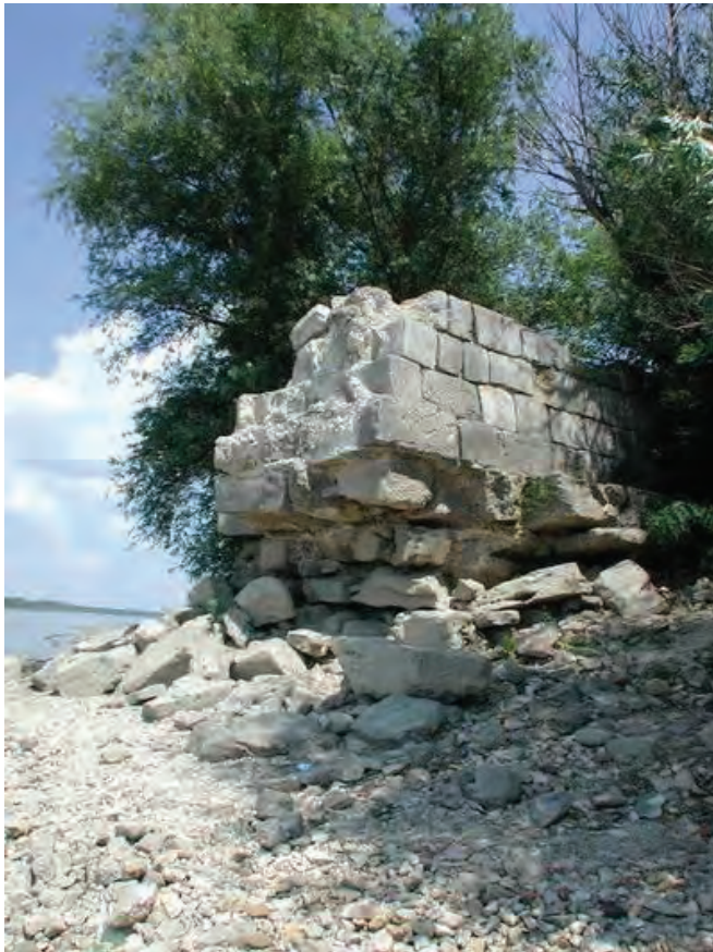
Fig. 2. Păcuiul lui Soare. The northern enclosure wall, destroyed by the waters of the Danube on the western side, 2000 campaign.
