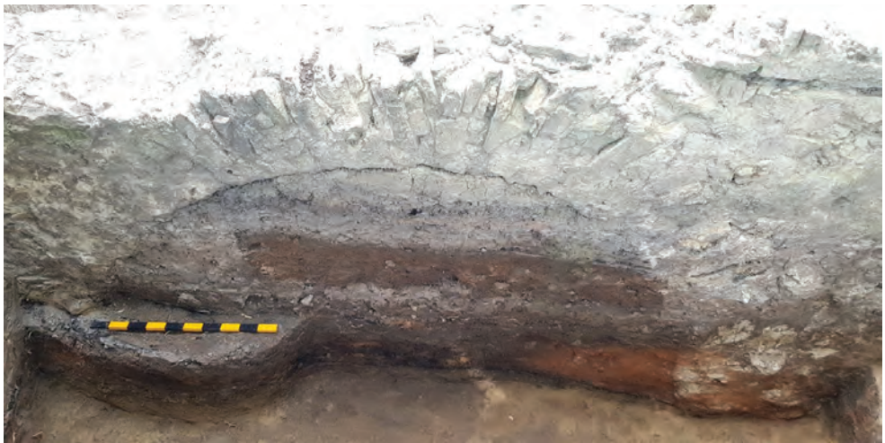
Fig. 3. 1–2 Images of the finds in excavation 2, features 94/96/108 (stages of research); 2 – Relieving arch built into the foundation on the eastern side of the building.
