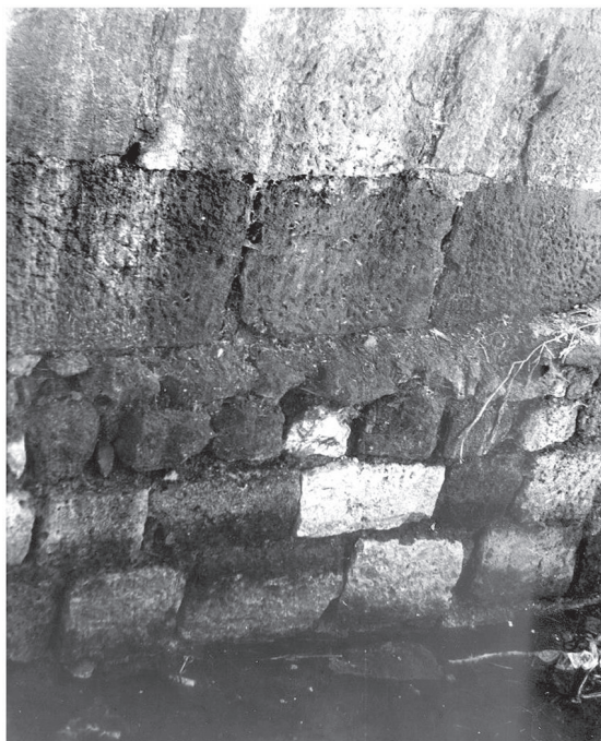
Fig. 5 - Section of the earlier fortress wall employed as a foundation for the 6 th c. fortification. Photo from the excavations of the eastern gates of Drastar.
